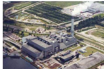
Advanced Flue Gas Cleaning
