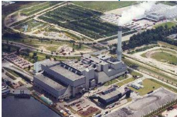
Advanced Flue Gas Cleaning
