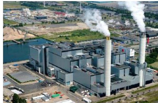
Waste-fired Power Plant (highest el. Efficiency world wide > 30%)
